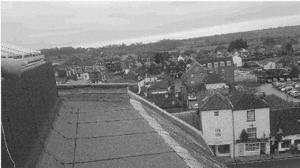
Figure 2: Wide view of the stone structure.
