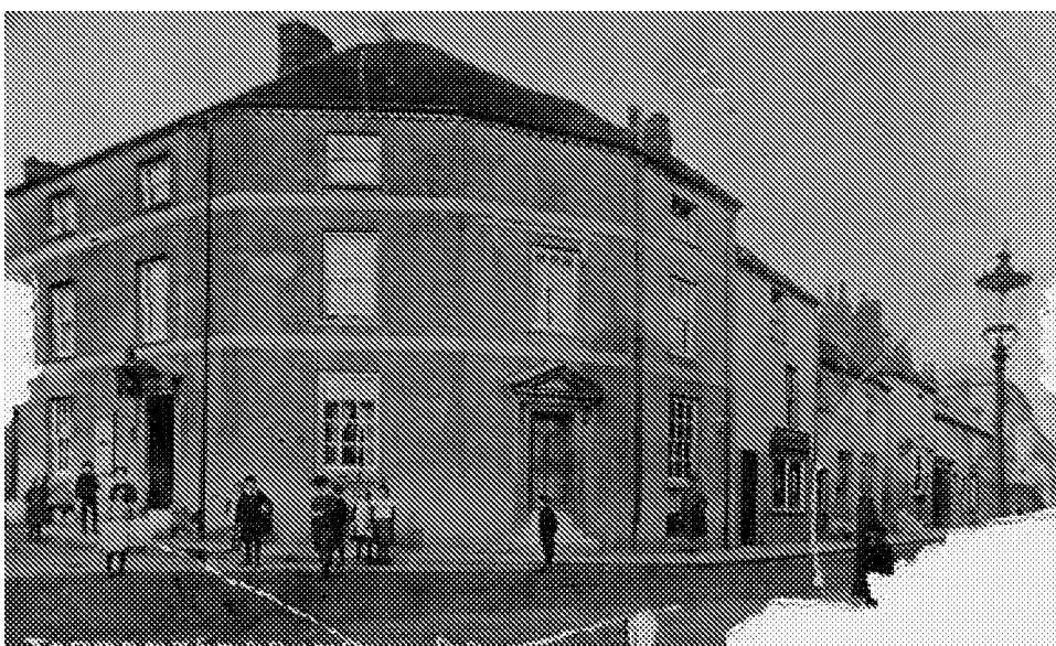
Figure 1. Application dwelling on left hand side with hood over front door. Photograph dates from 1914.
