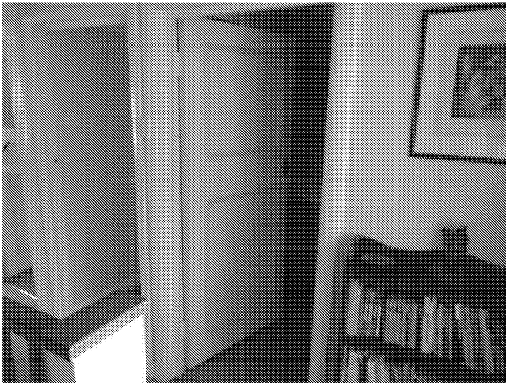
Figure 12. Door to be blocked-up on top floor.
