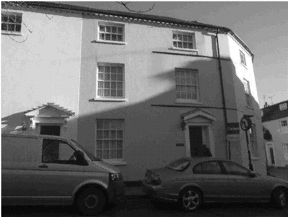
Figure 2. The frontage to School Lane.
