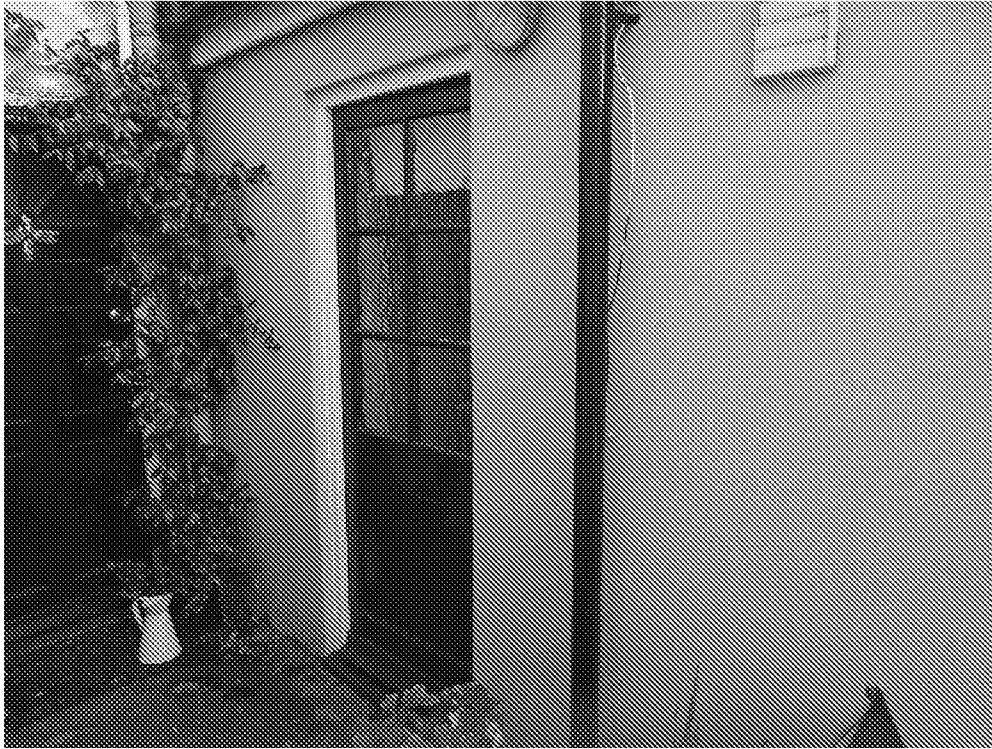
Figure 3. Existing back door.
