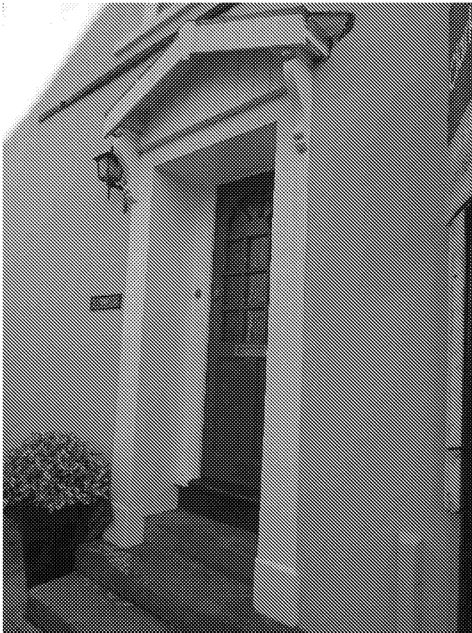
Figure 4. Existing front door and surround.
