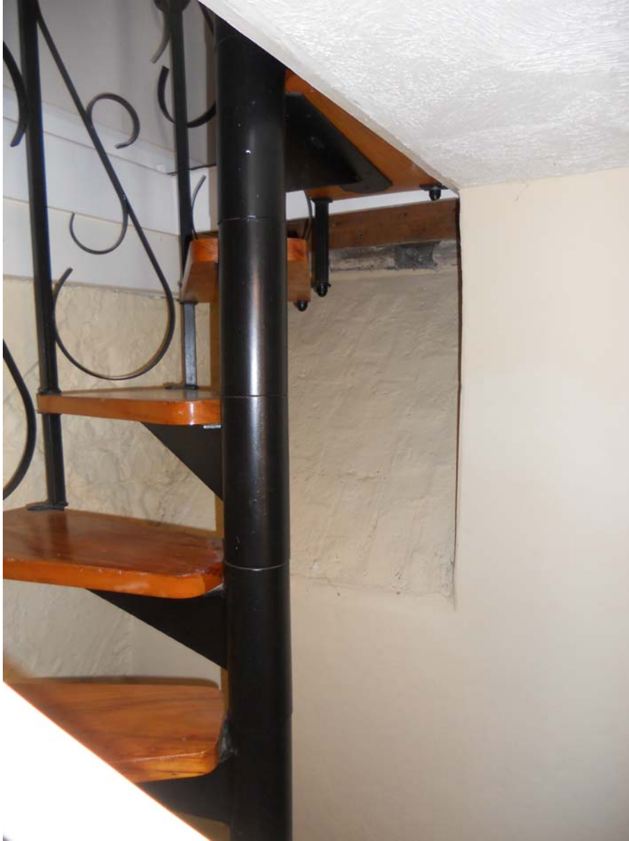
View P 02 (Cellar)
