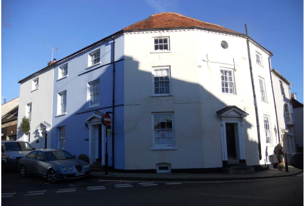
Photograph of Property at the Junction of Tarrant Street and School Lane
