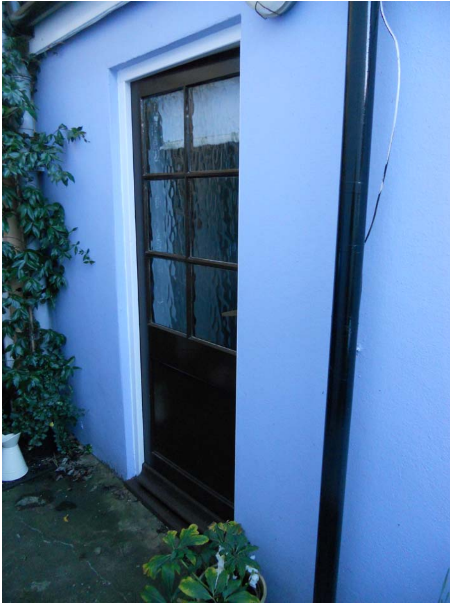
Rear External Kitchen Door
