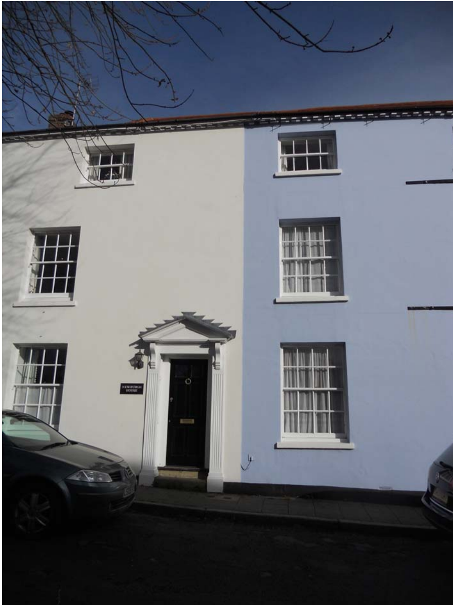
Front Elevation of Newburgh House (adjacent property)
