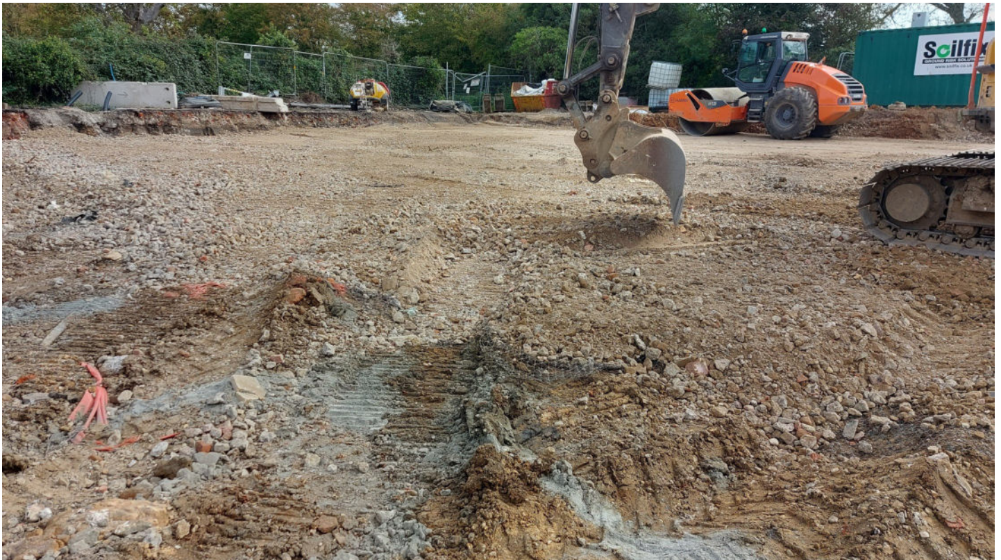
Photo 3. Pile Mat at 2.1m AOD looking East 29/09/2023
