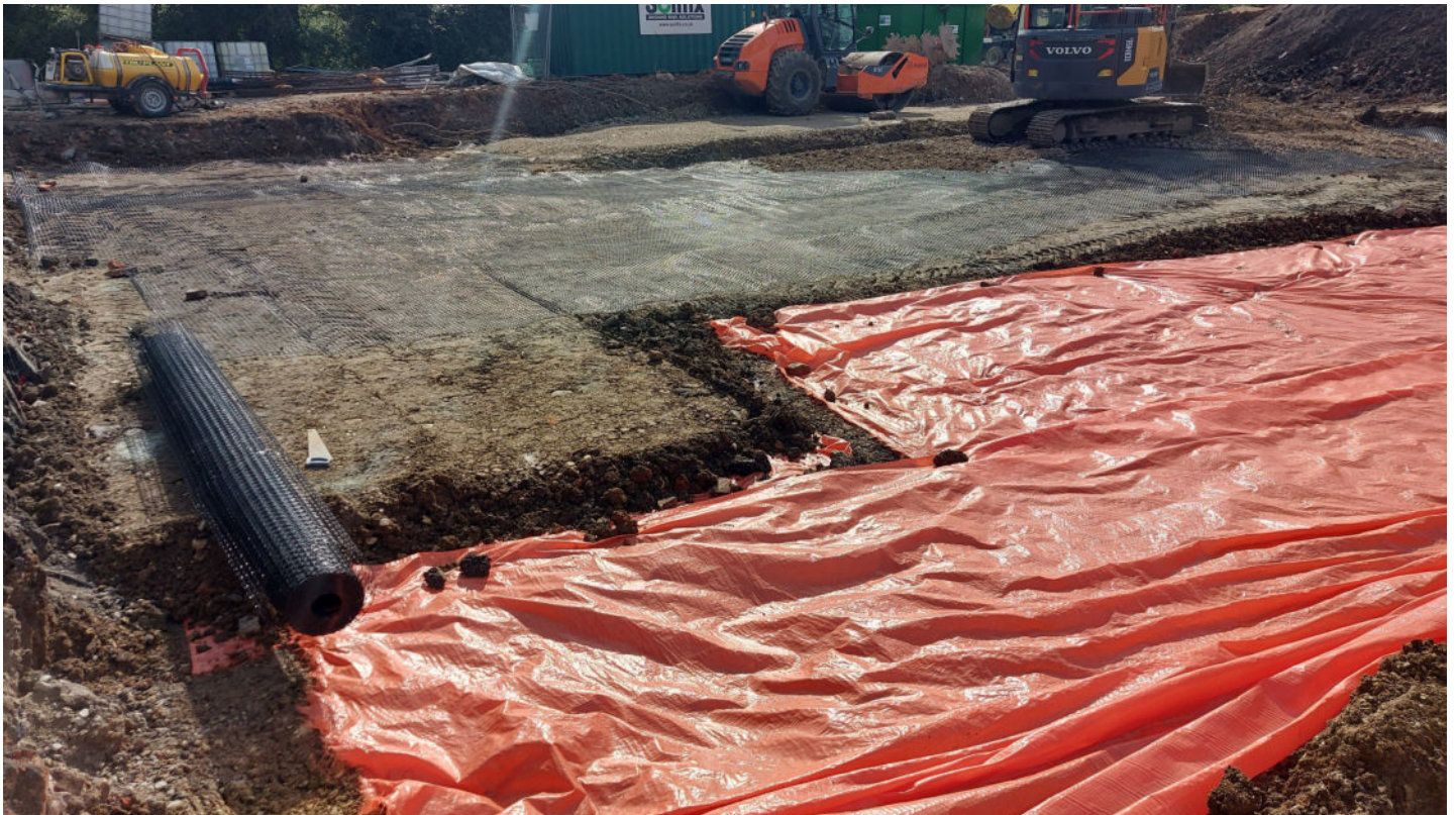
Photo 1. Pile Mat construction progress Cell F7 29/09/2023 AM
