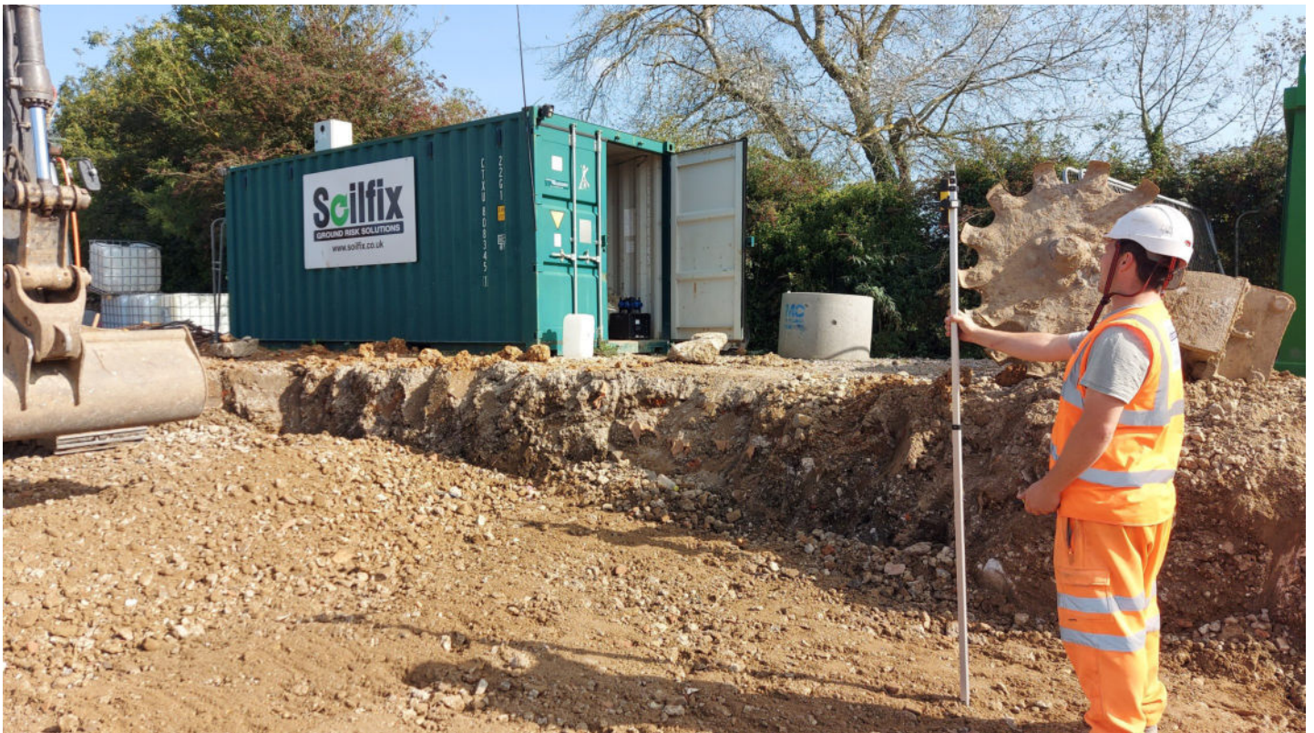
Photo 2. Pile Mat construction progress Cell F6 29/09/2023 AM
