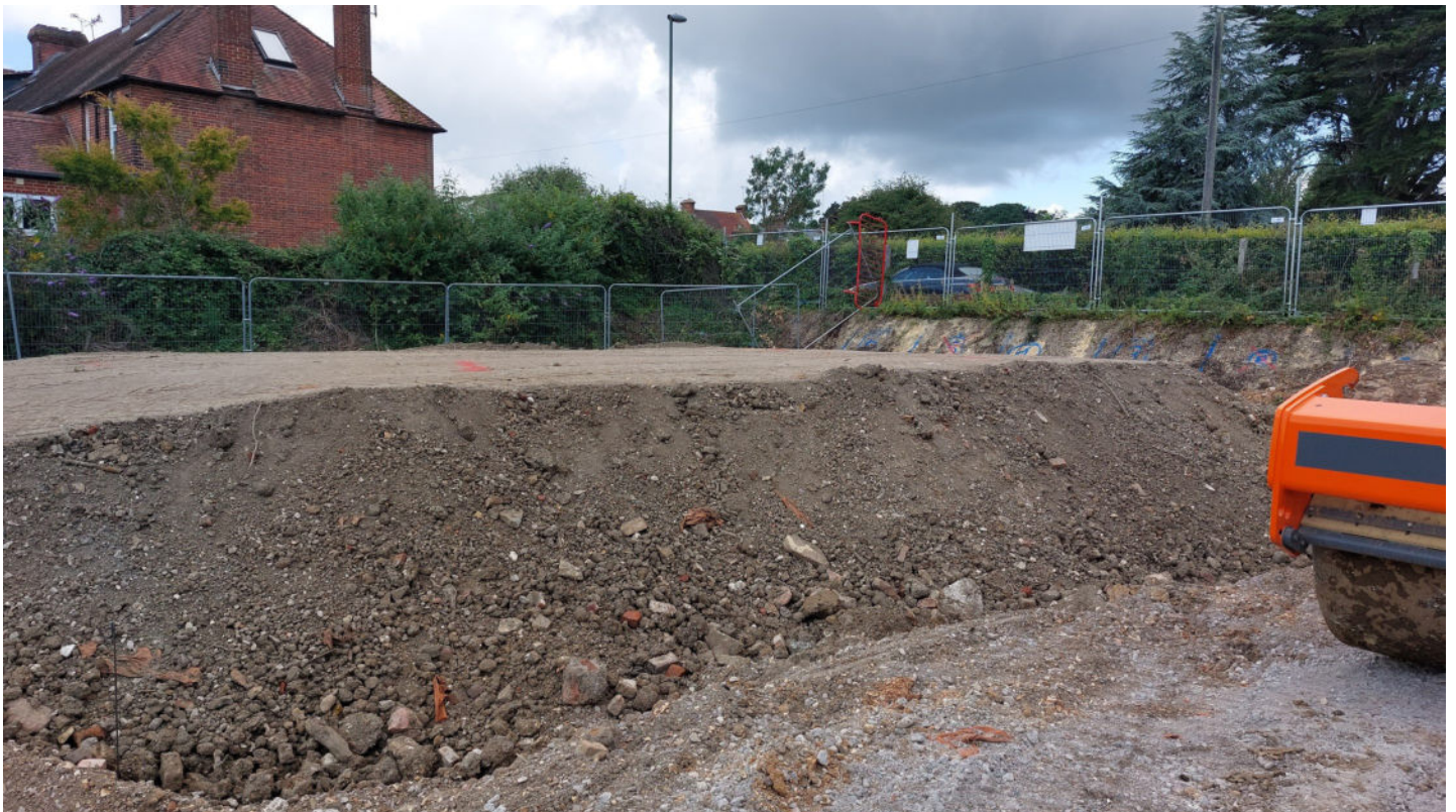
Photo 2. Pile Mat Cell B1 August 2023.
