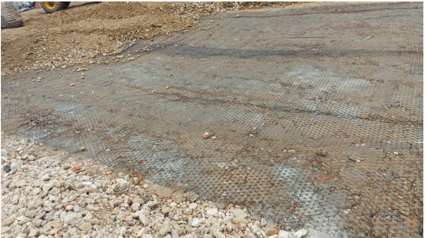
Photo 4. Pile Mat at 2.1m AOD looking North 02/10/2023
