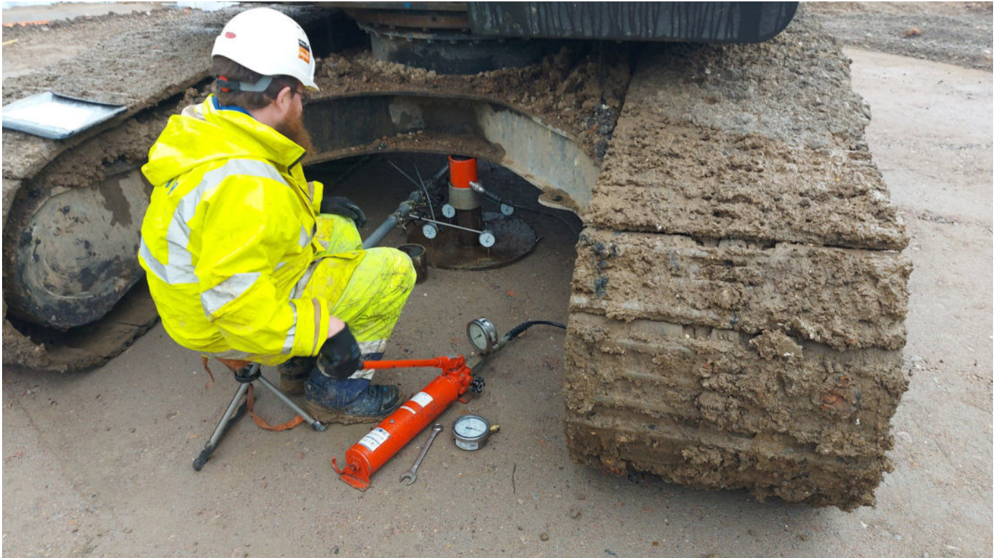
Photo 1. Plate load test 18th August 2023.
