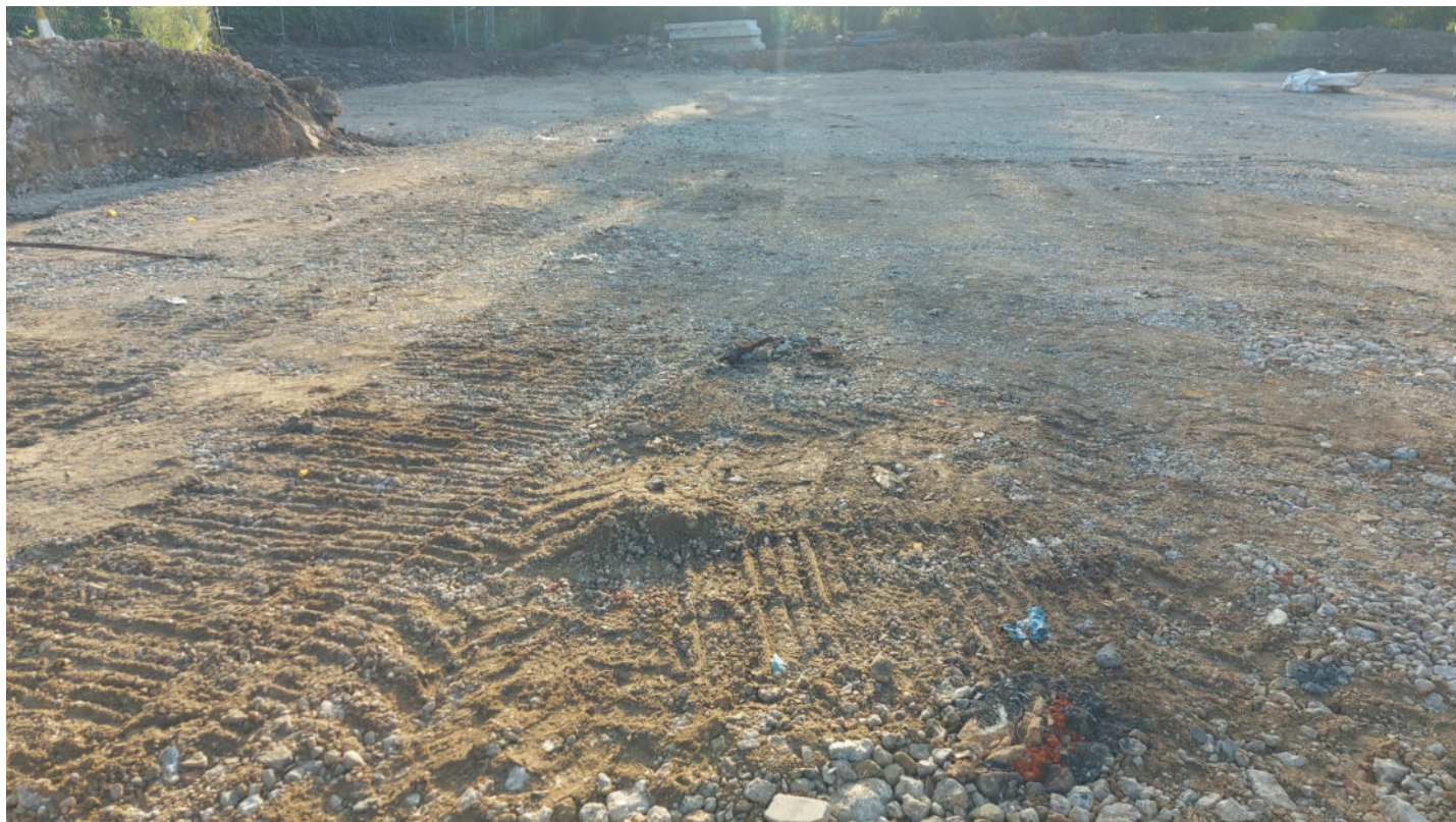
Photo 5. Pile Mat at 2.1m AOD looking South East 03/10/2023
