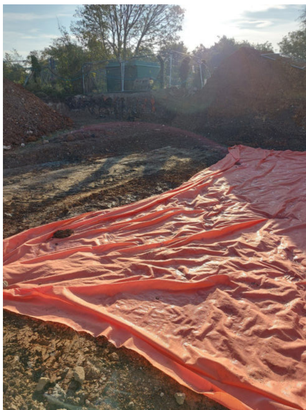
Photo 6. Lower mat geo marker
