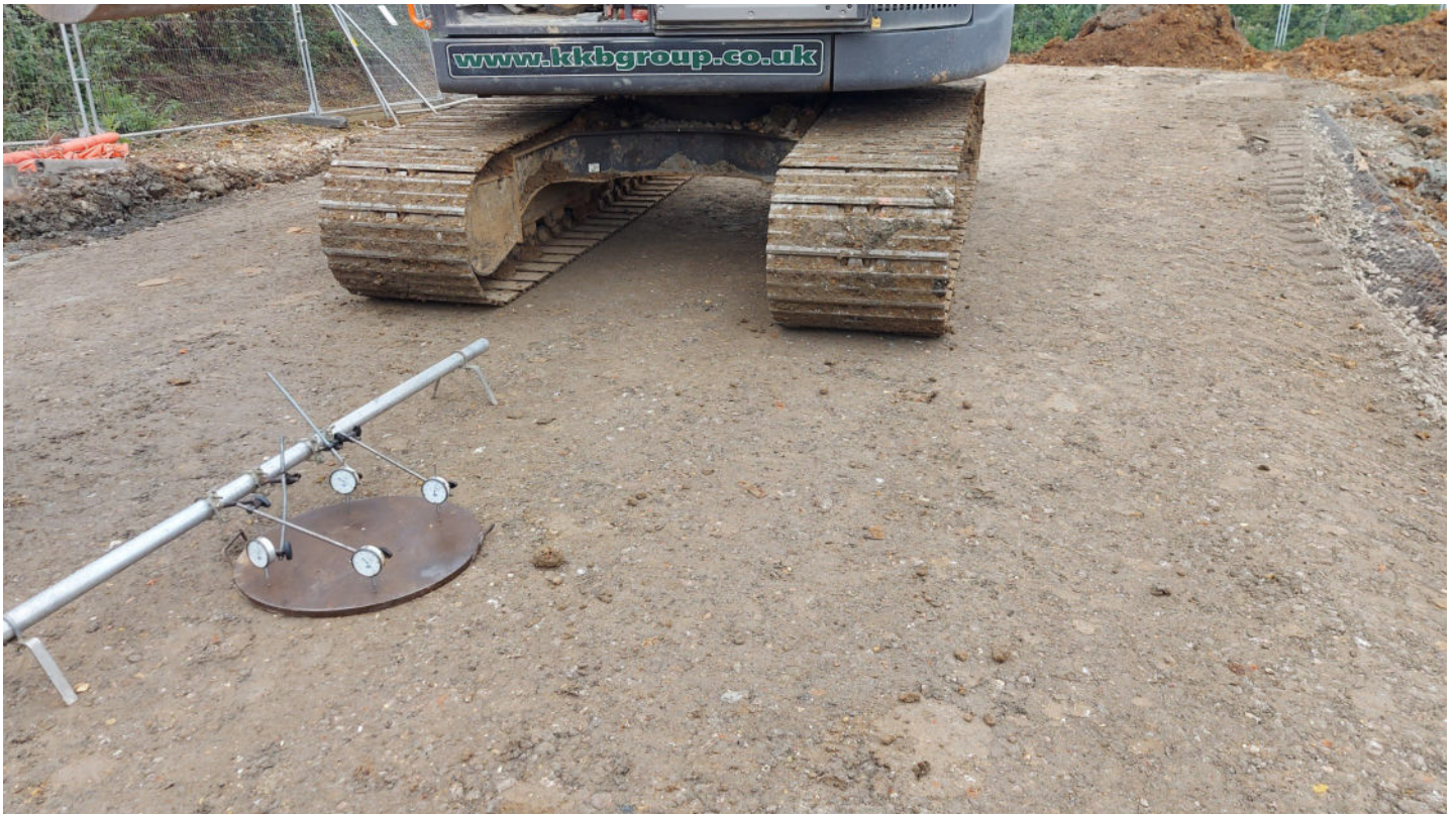
Photo 9. Transition Ramp with plate test being set up (19/09/2023).
