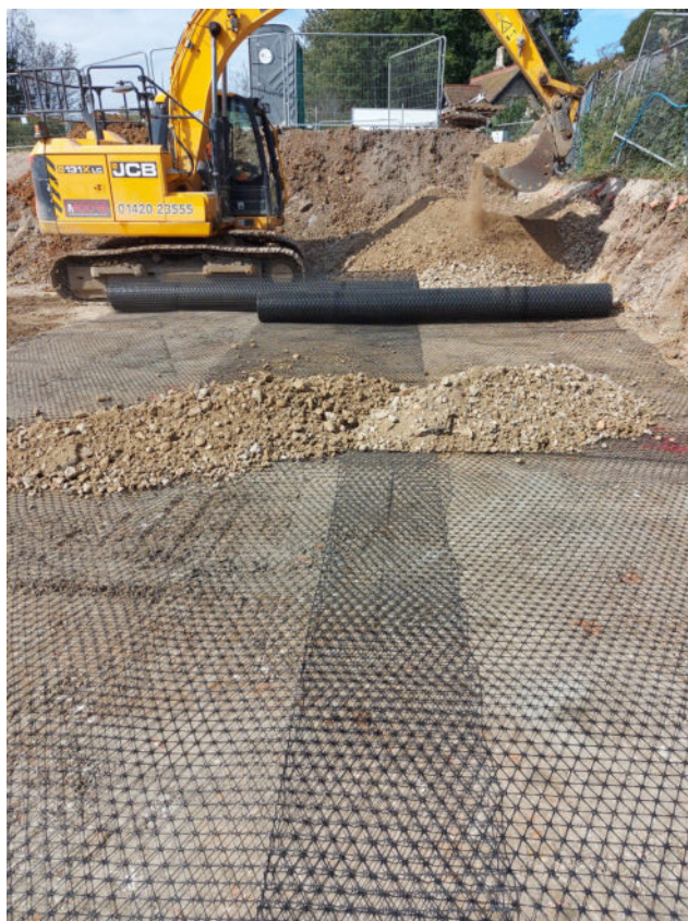
Photo 8. Lower mat geogrid
