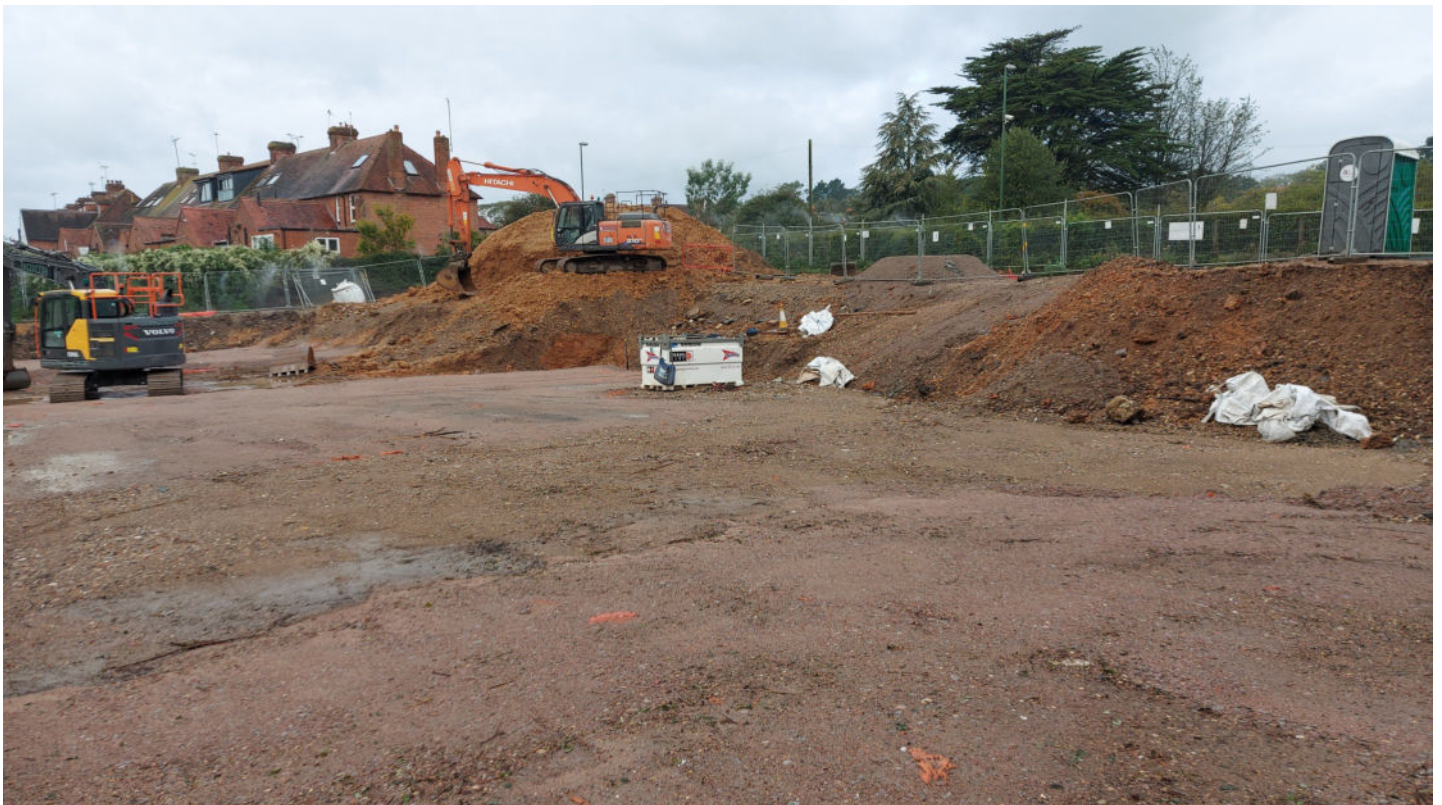
Photo 4. Pile Mat Cells D3 to F4 with entrance ramp (18/09/2023).
