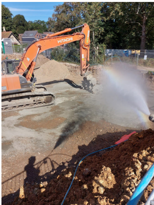
Photo 7. Lower mat cement stabilisation
