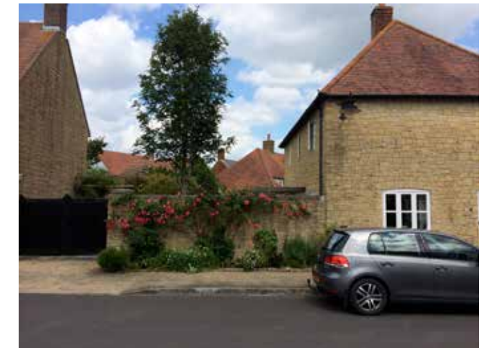
Boundary walls enhance enclosure
