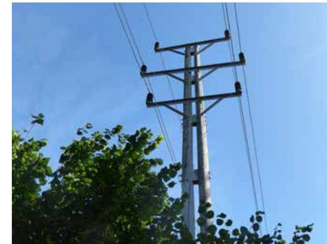
View 11 - Existing overhead electricity power lines
