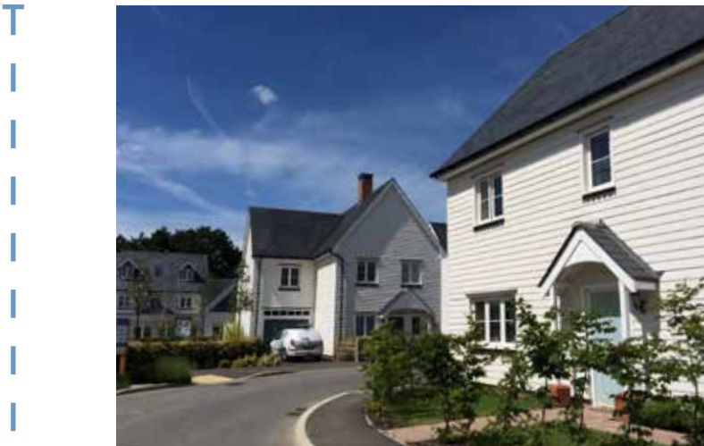
Weather boarding on detached properties
