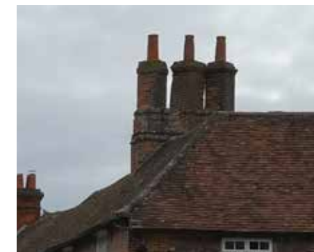
Brick chimney stacks
