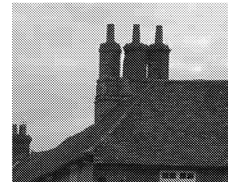
Brick chimney stacks
