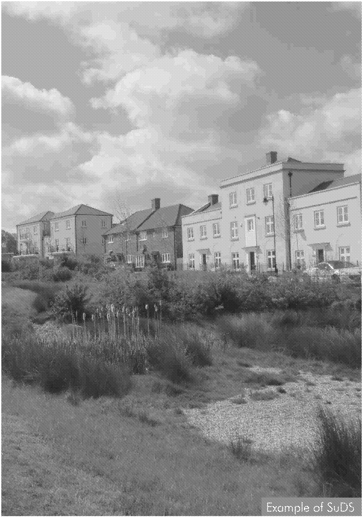
Example of SuDS
