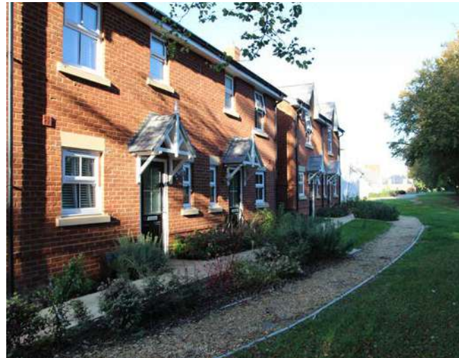
Terrace housing overlooks site boundary
