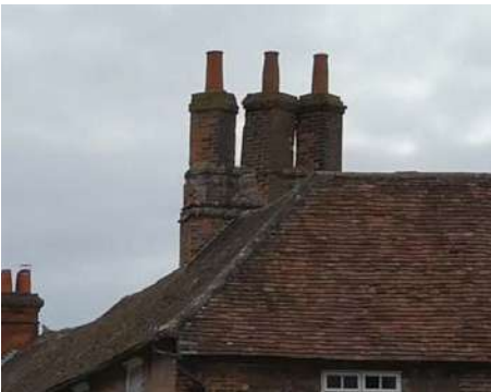
Brick chimney stacks
