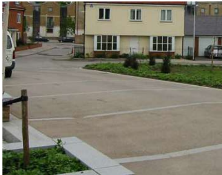
Bound coloured asphalt
