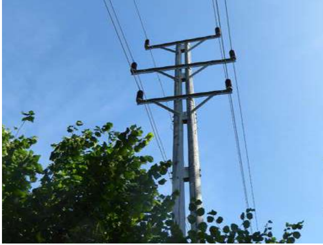
View 11 - Existing overhead electricity power lines
