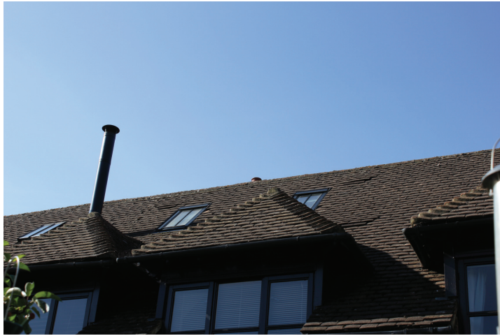
Fig 01 No. 9 and 10 Old Poor House
