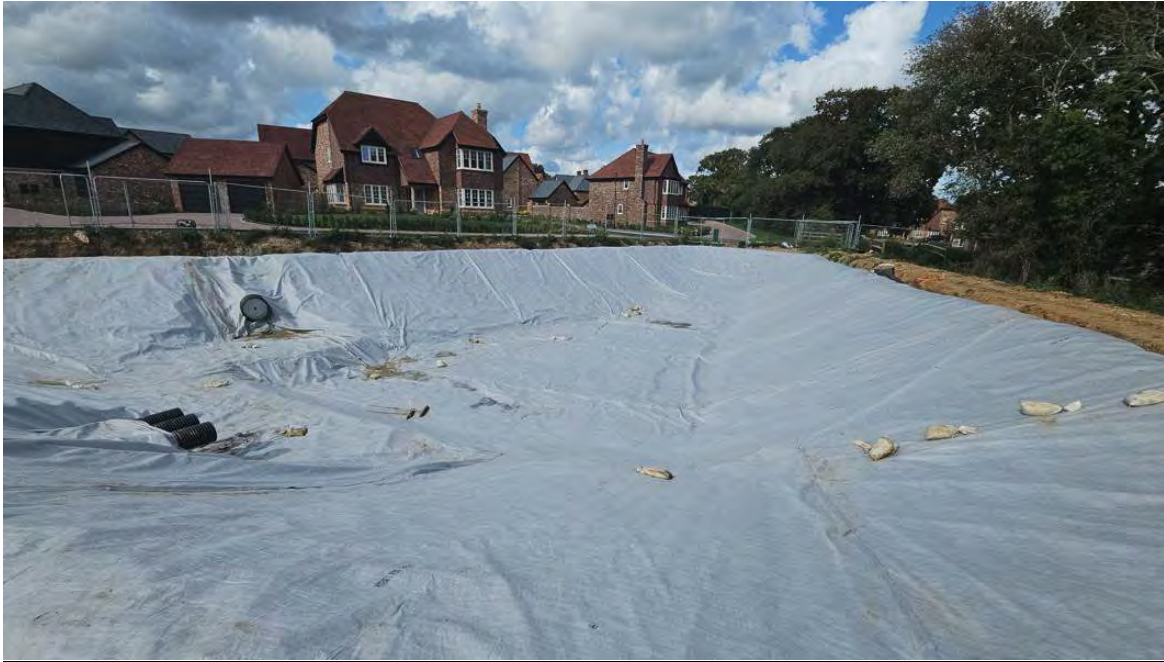
Figure 6 – Pond 2 Liner Installation
