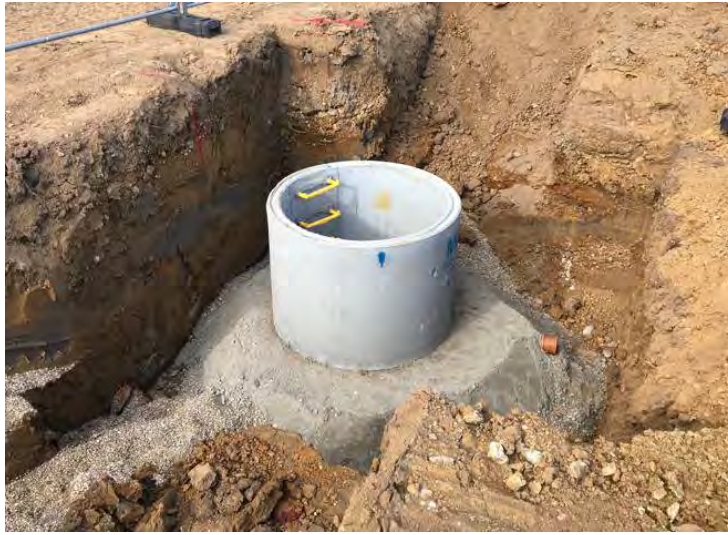
Figure 1 – Pre Cast Concrete Manhole
