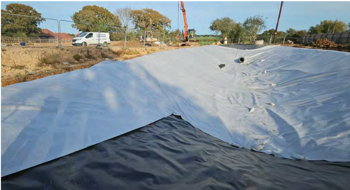
Figure 7 – Pond 3 Liner Installation
