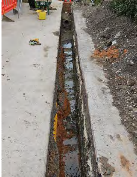
Figure 4 – Rising main trench construction
