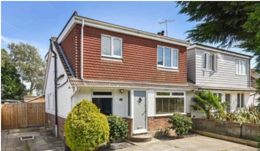
The cottage as viewed from the south
