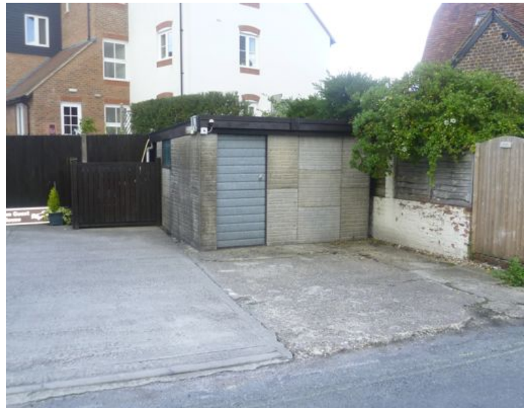
Existing concrete panel Garage to be removed
