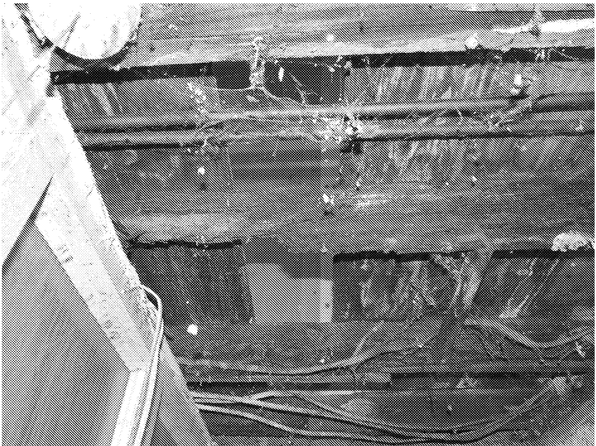
First floor joist damage
