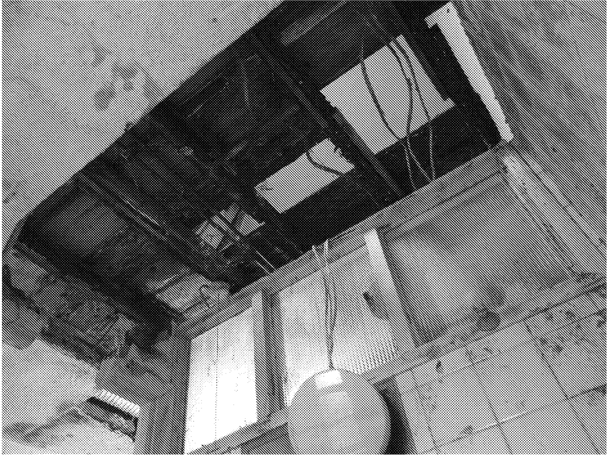
First floor joist damage
