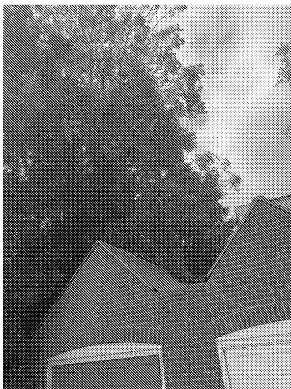
Figure. 7 Ash and Bay tree over garage roof (T3 & T4)
