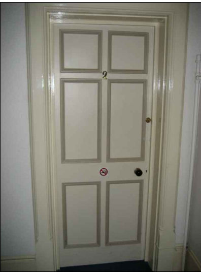
Existing Bedroom 2 6-panel Door.
