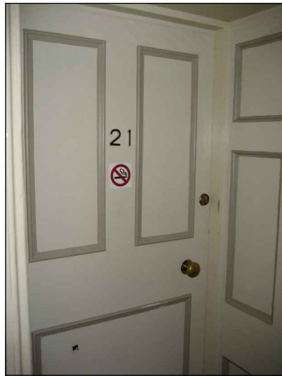
Existing Bedroom 21 Door with applied beading.
