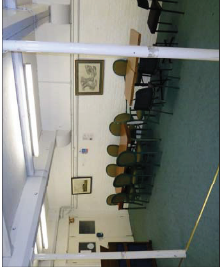
Lower Ground floor meeting room area - showing cast iron posts and infill to external arches where brickwork and windows are to be removed and new glazing screens installed in historic open arches
