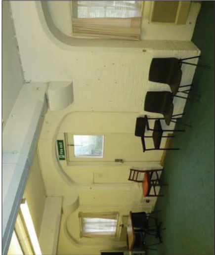
Lower Ground floor meeting room area - showing cast iron posts and infill to external arches where brickwork and windows are to be removed and new glazing screens installed in historic open arches
