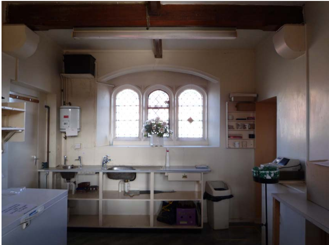
This opening is considered to be of low historic merit in the overall context of the building, given that it is a simple flat headed lintel of later insertion.
