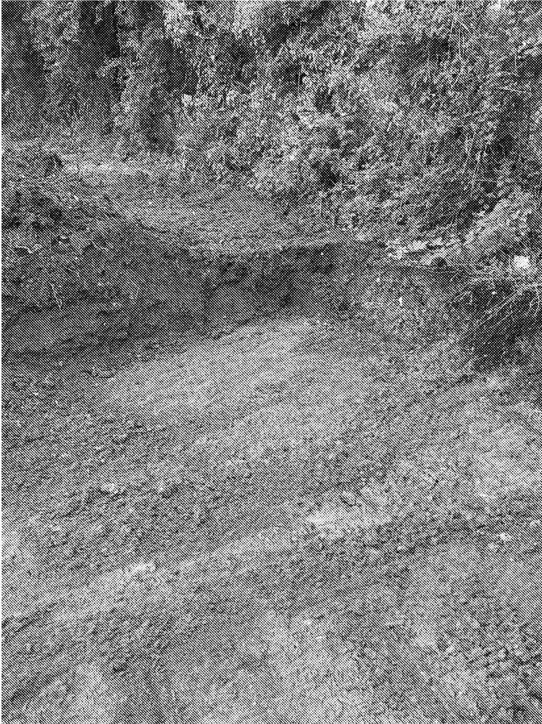
Plate 26 – Excavating to natural ground in Area 2
