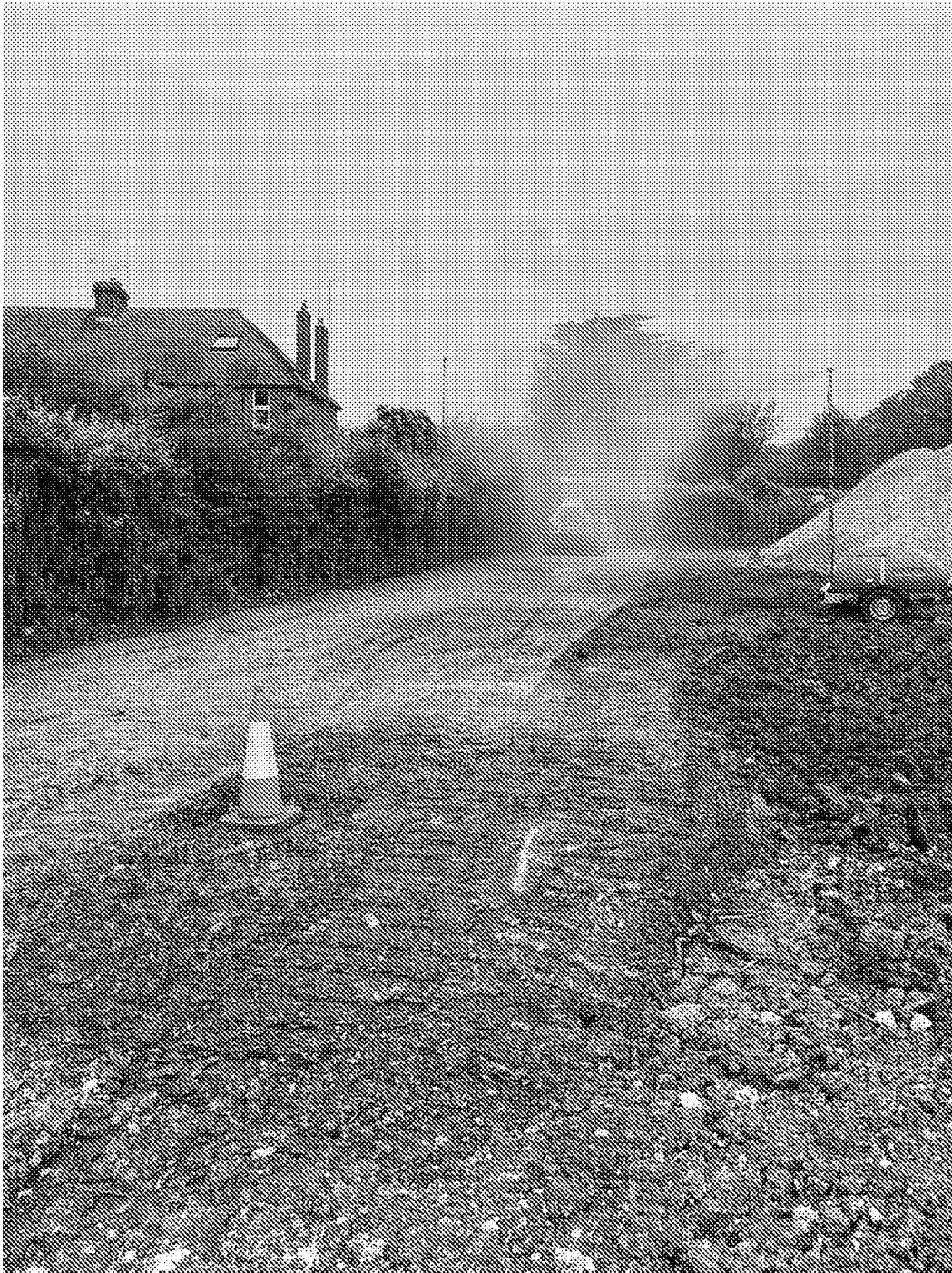
Plate 27 – Re-compacting the made ground in Area 2
