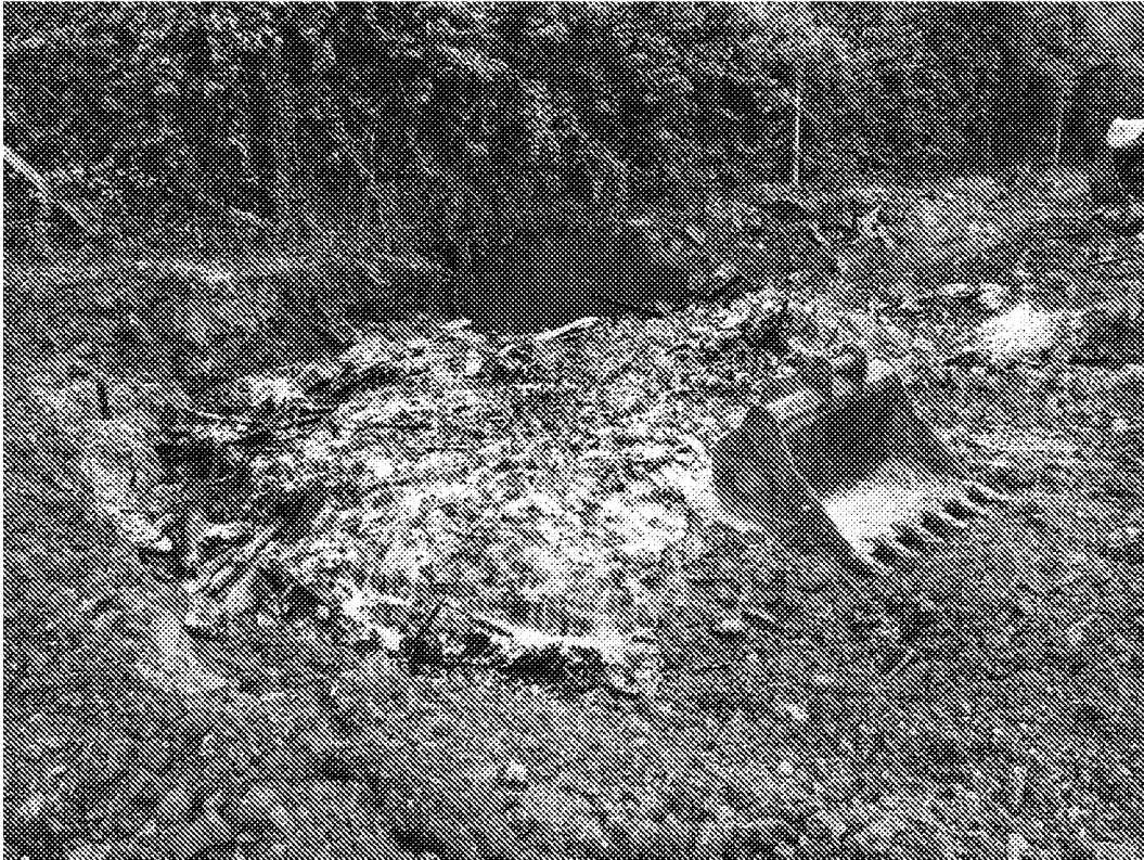
Plate 37 – Contaminated materials within former gasholder (feature no. 4)
