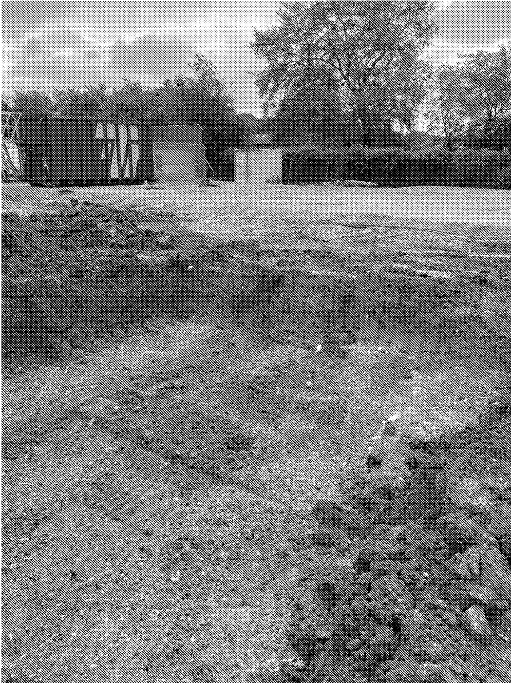
Plate 32 – Excavation to natural ground in grid C5
