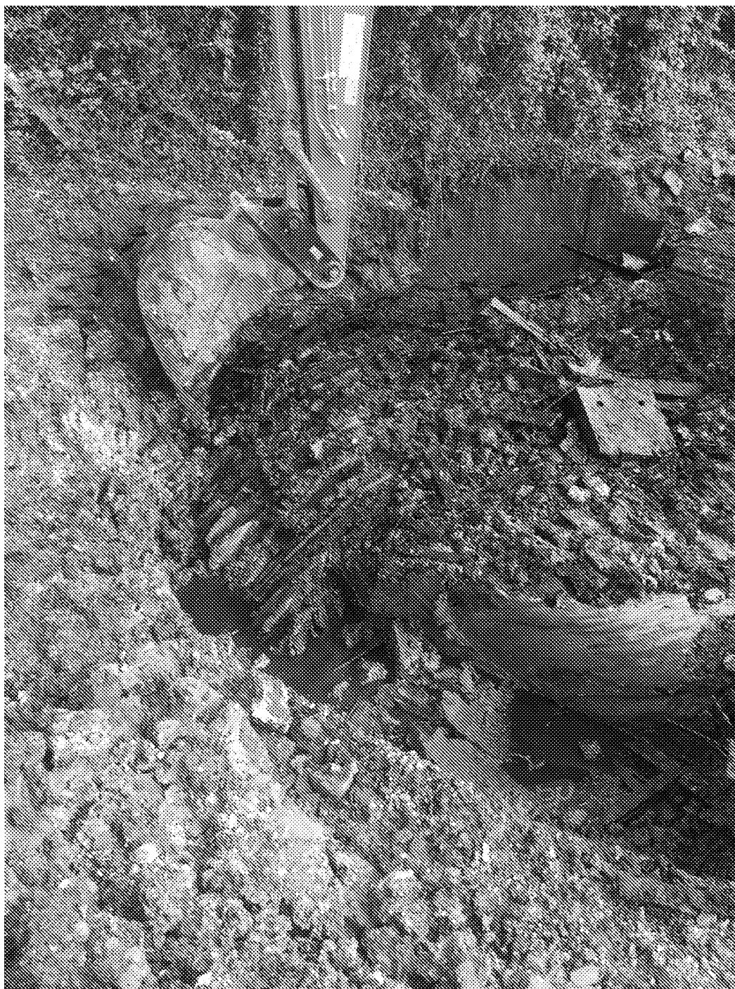
Plate 38 – Excavating contaminated materials within former gasholder (feature no. 4)
