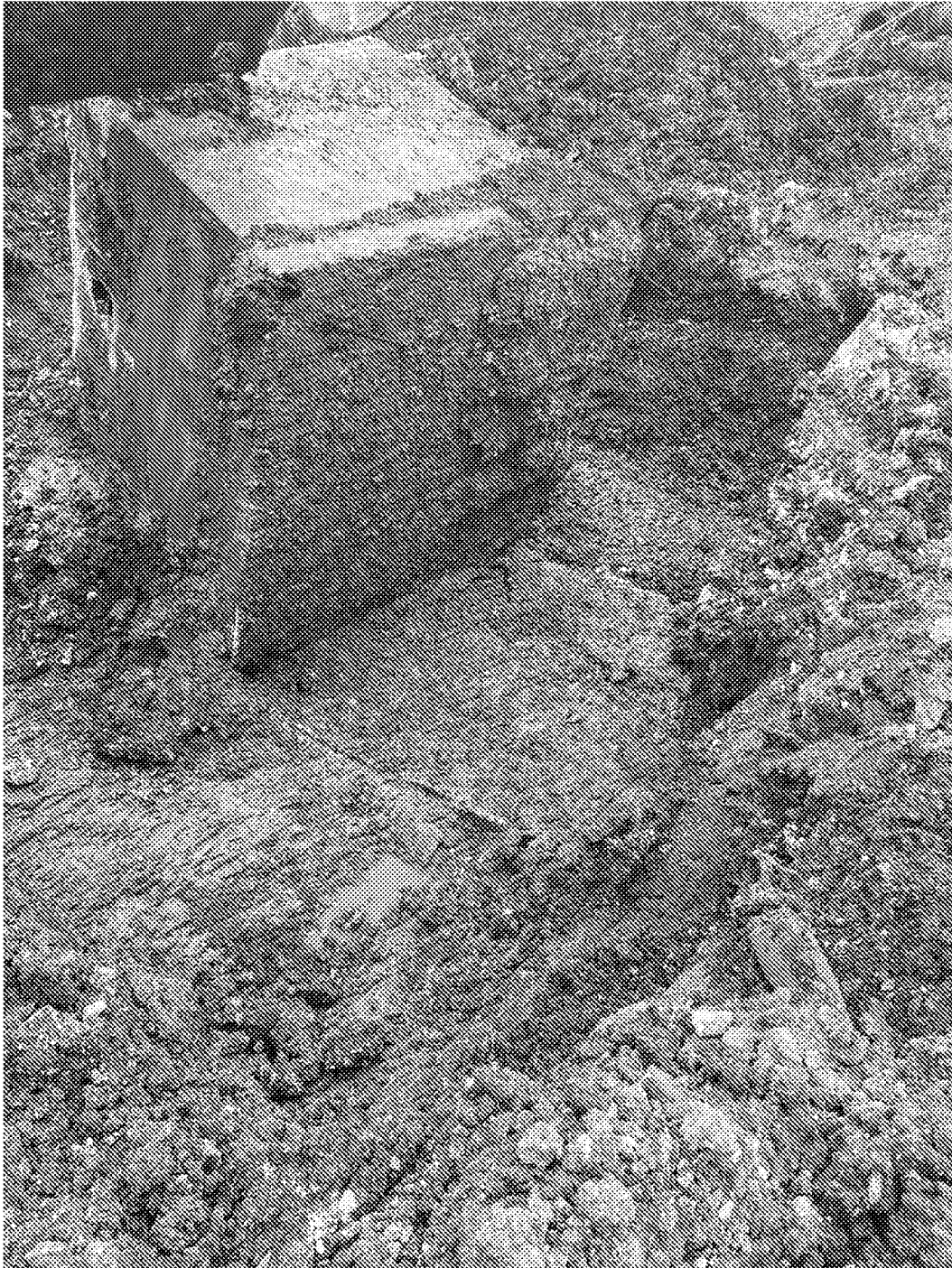
Plate 15 – View of further concrete chambers being removed
