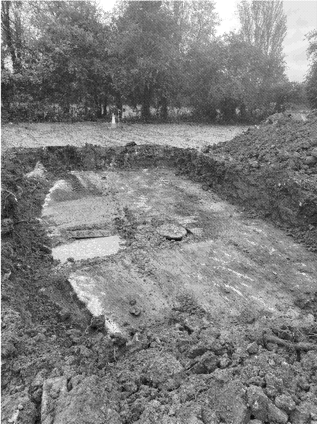
Plate 23 – Exposing the gas holder base across grid B7/C7
