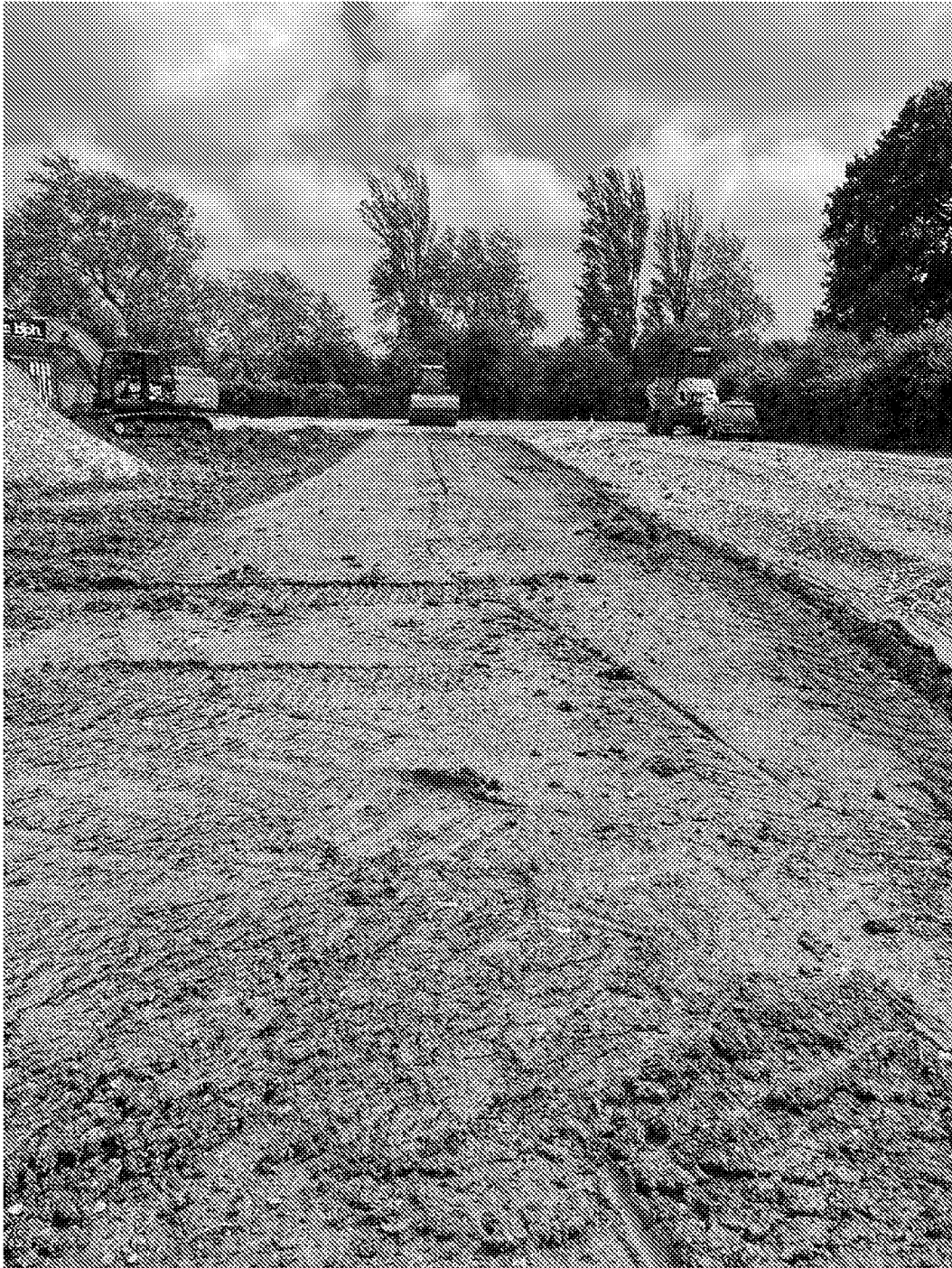
Plate 34 – Re-compacting made ground across Area 3
