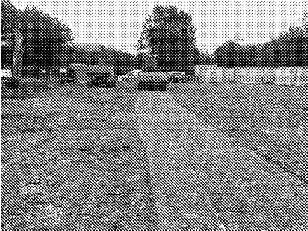
Plate 25 – Capping layer placed across Area 1
