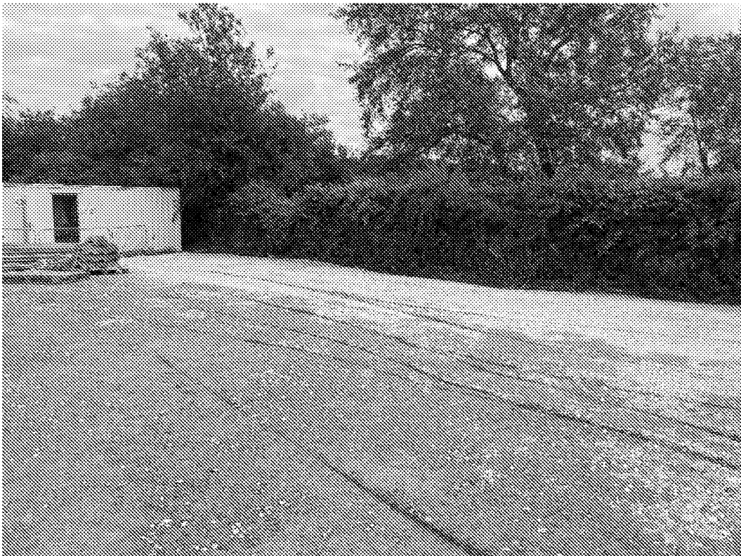
Plate 25 – Capping layer placed across Area 1
