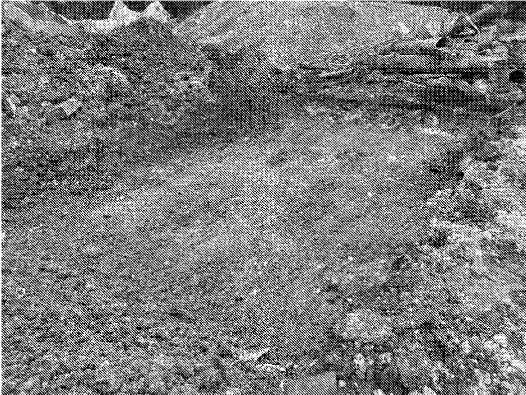
Plate 19 – View of natural soils encountered following made ground removal (Grid D6)
