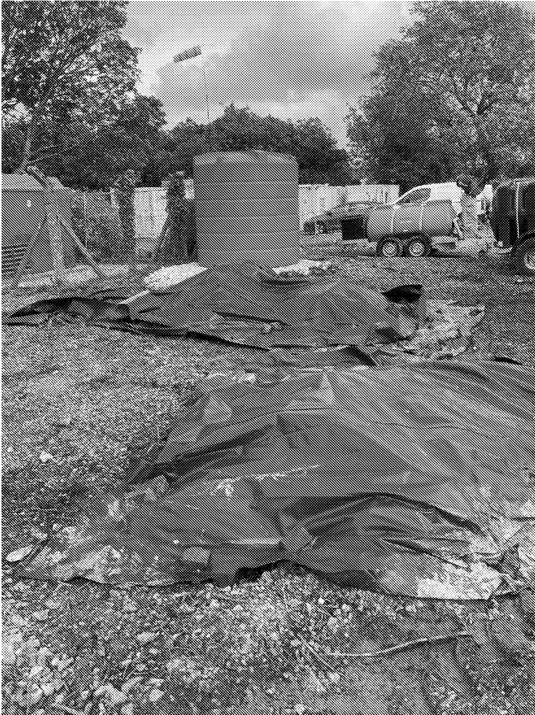
Plate 31 – Segregation of small amounts of contamination encountered from Areas 1-3
