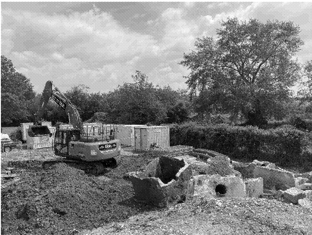
Plate 17 – View of concrete chambers following removal in Area 1
