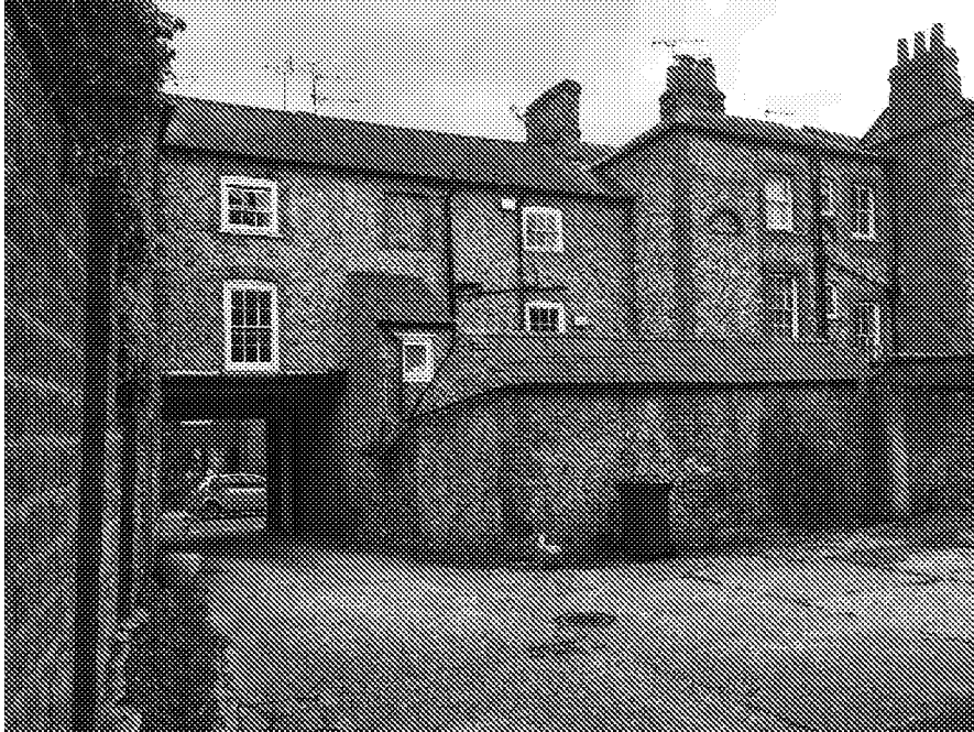
Figure 4: Rear facade of Tarrant Street Houses and access to Yard
