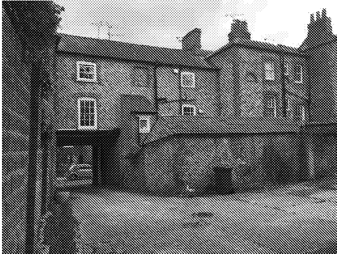
Figure 7: Rear façade of Tarrant Street Houses and access to Yard
