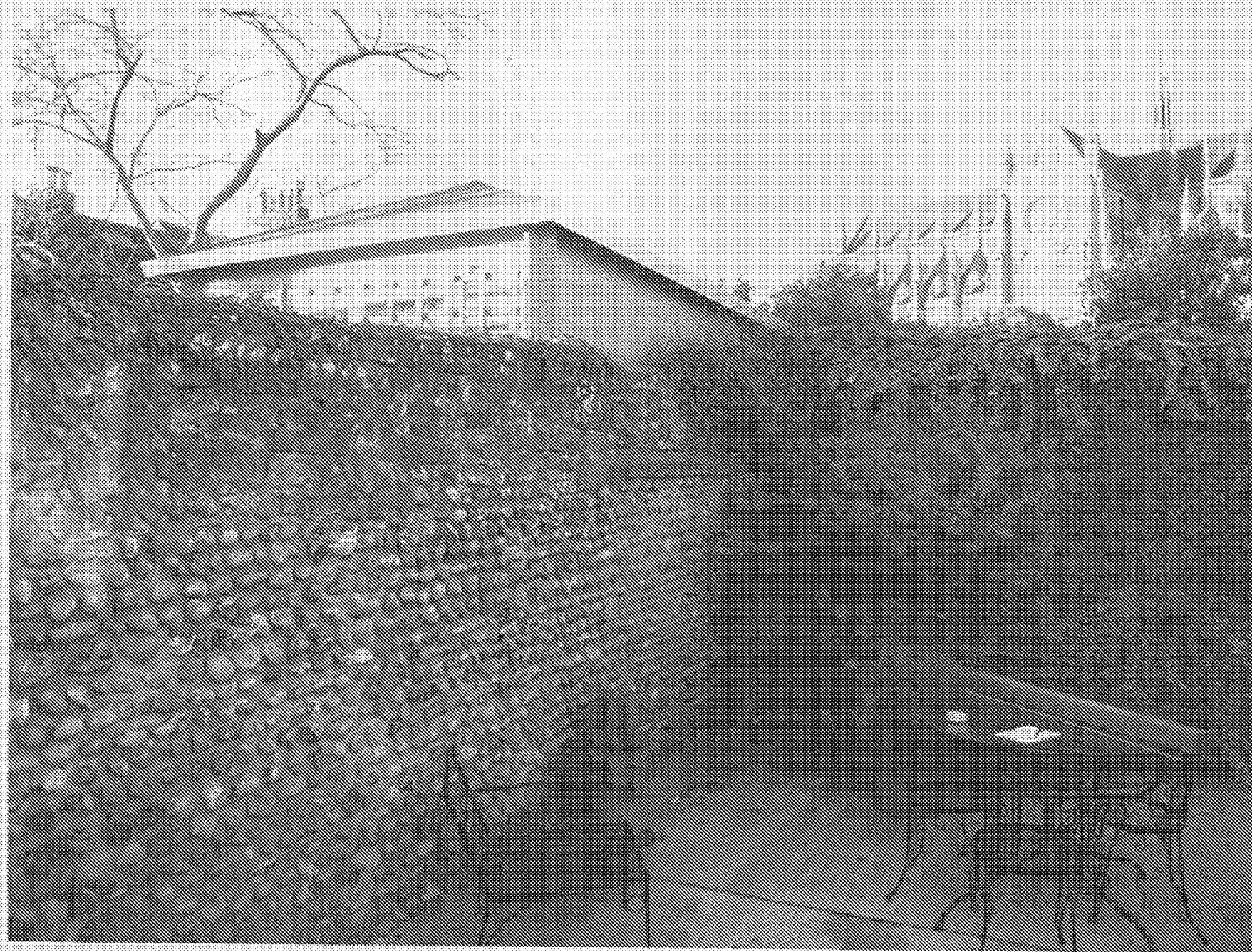
PHOTO No 1 "VIEW OF NEW 206 CABIN FROM BACK GARDEN" AB/10/15/HH
