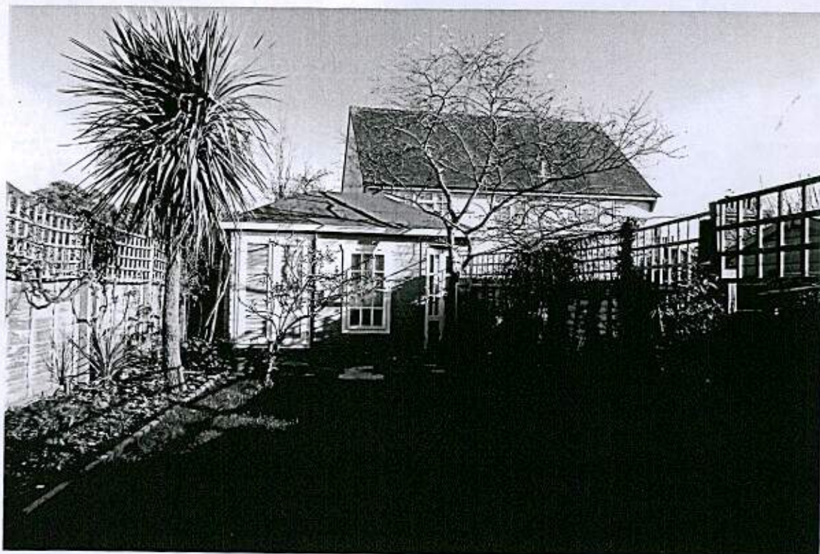
STRUCTURES AFTER 24TH SEPTEMBER 2014
