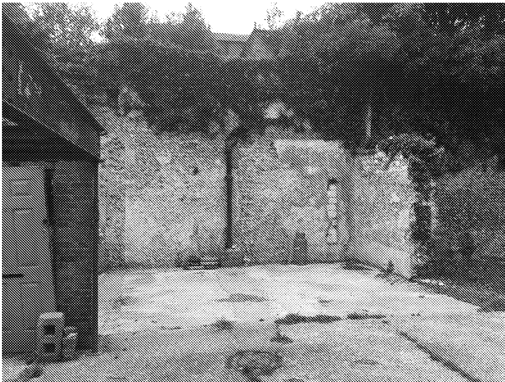
Figure 11: Wall at back of site (boundary wall to garden of 61 Maltravers Street)
