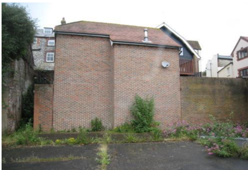
Photograph 6 - View looking north towards the north western corner of the site
