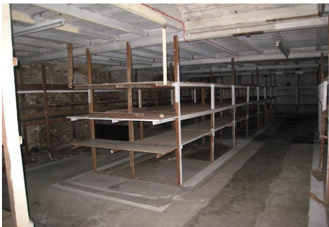
Photograph 13 - View looking west inside the most westwards part of the warehouse
