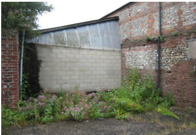
Photograph 7 - View of the location of the former above ground diesel tank
