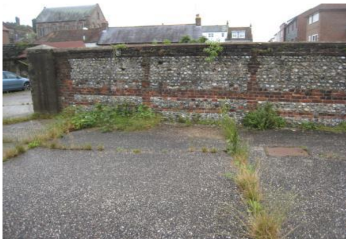
Photograph 8 - View of the position of the former buried petrol tank
