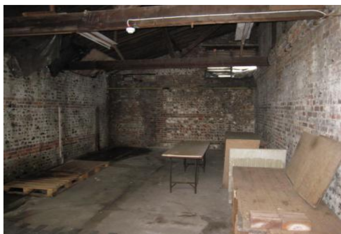
Photograph 12 - View inside the southern most warehouse room
