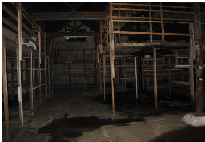
Photograph 14 - View looking north within the northern most warehouse building
