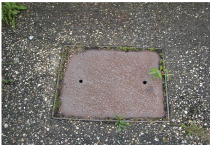
Photograph 9 - View of the cover of the former buried petrol tank
