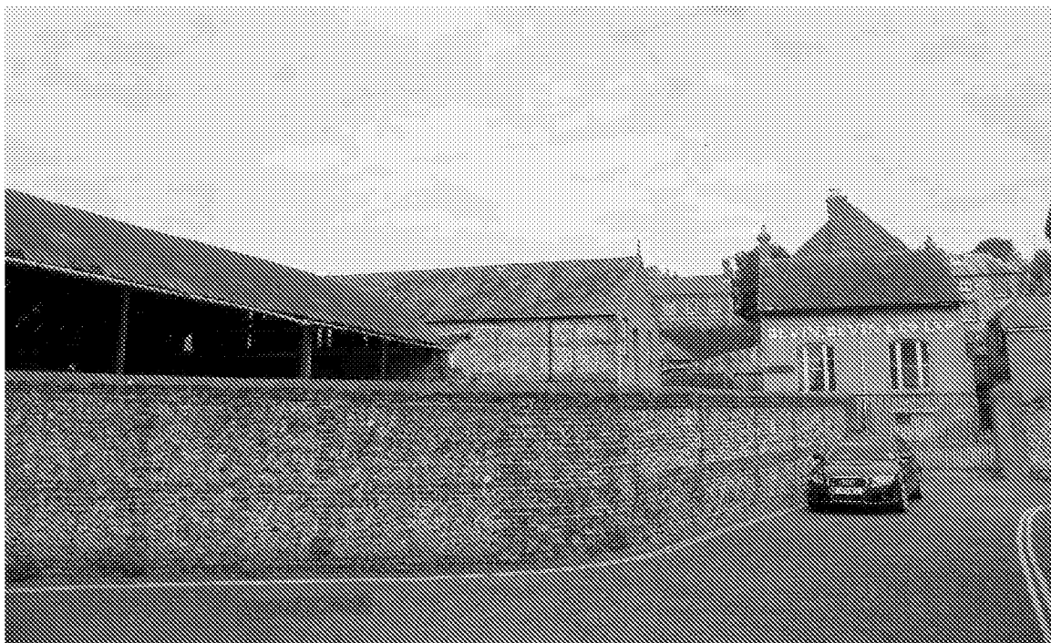
Figure 17a and b: Sections of boundary wall –south (above) and south-east boundary (below) - collectively described as Building 13
