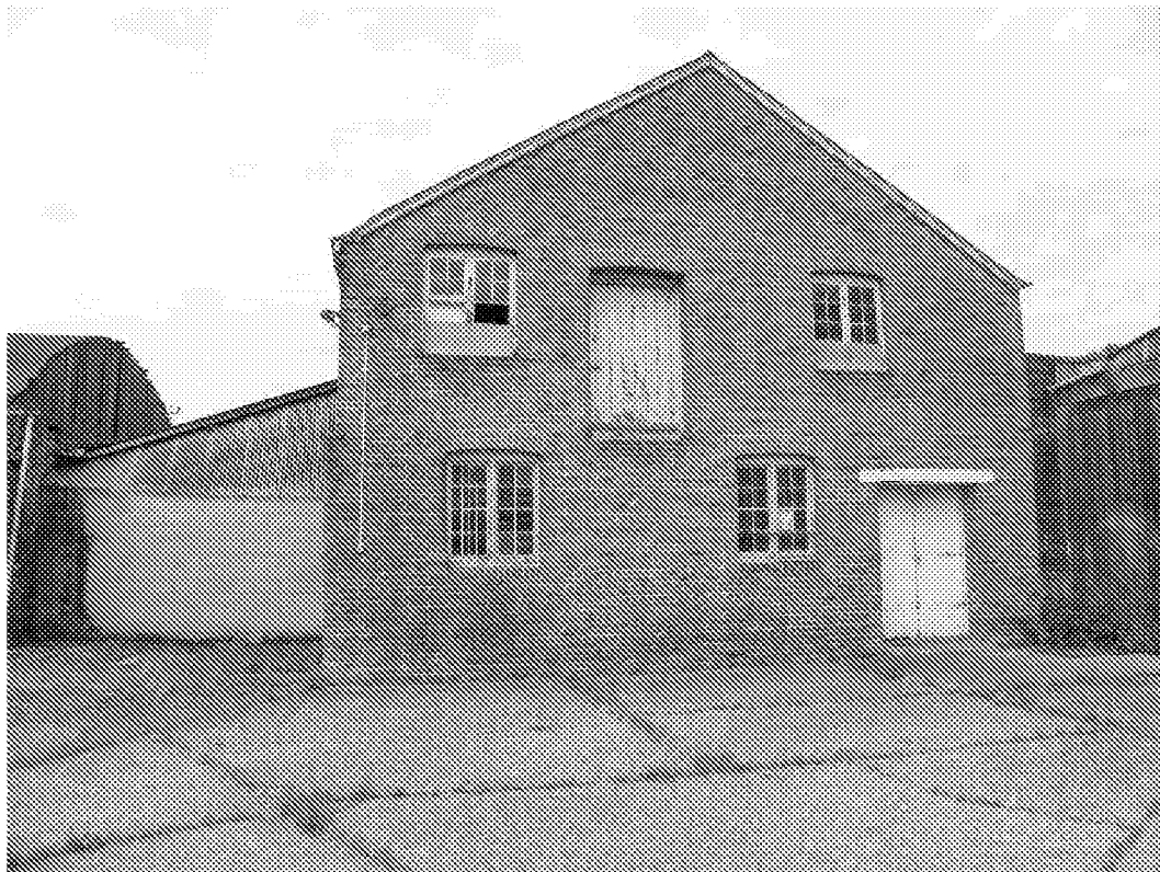
Figure 13: East elevation of Building 9
