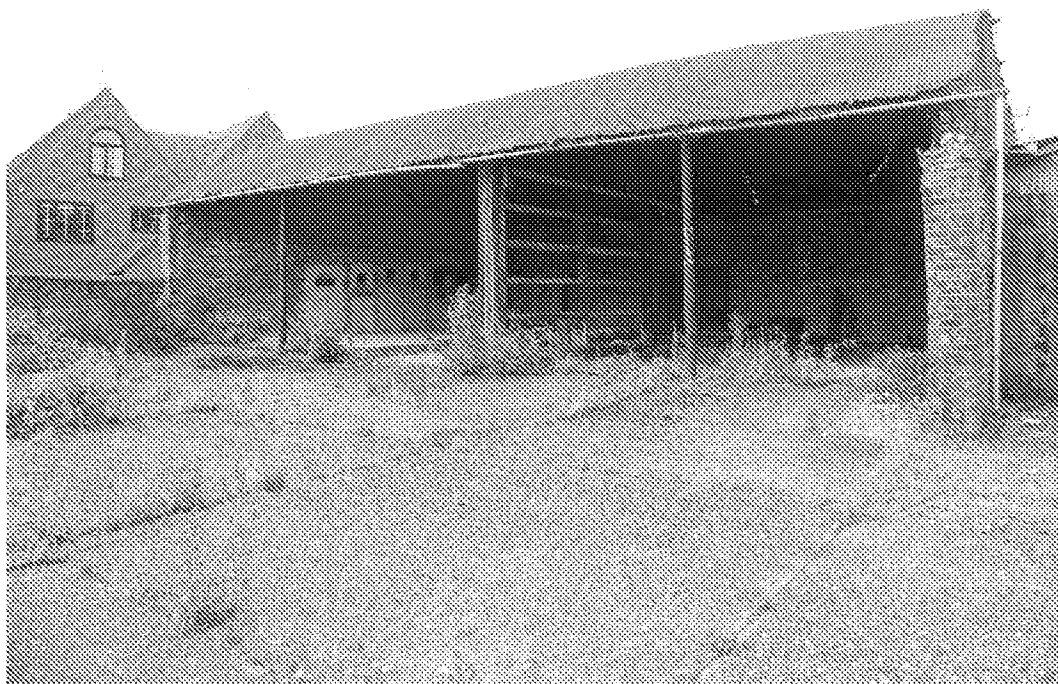
Figure 15: East and south elevation of Building 11
