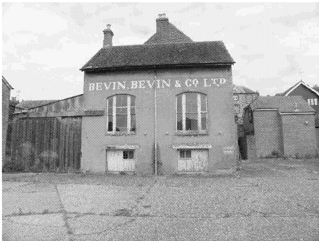
Figure 4: South elevation of Building 2
