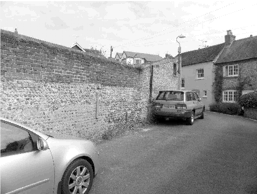
Figure 17c and 15d: Boundary walls (Building 13) south-eastern to east of entrance (above) and eastern boundary of the site (below)
