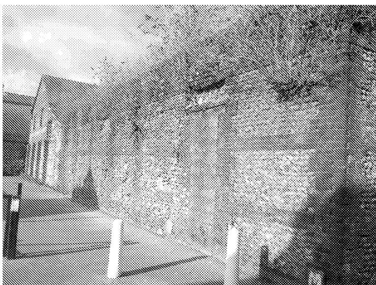
Figure 2 - West wall of Building 13 showing vegetation growth and loss of masonry facing
