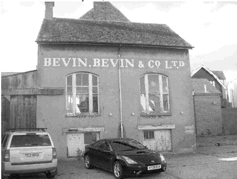
Photograph 2.2: View of the building to the south of the Grade II listed building, Bevin & Bevin Brewery Site, Arundel.
