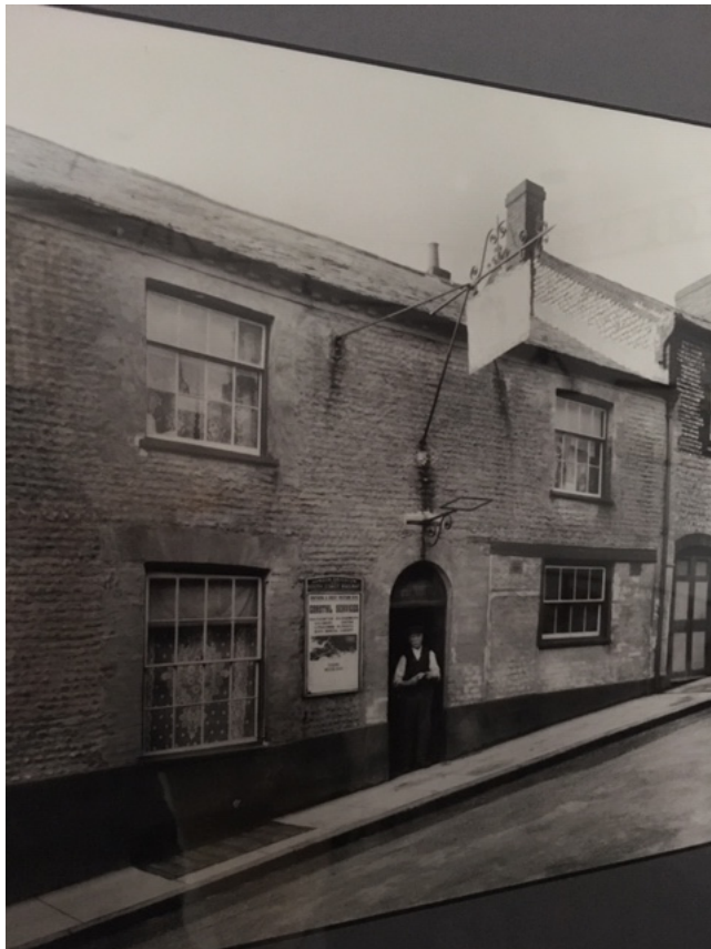
Photo – The Old Ship – property is to the right of the gentleman in the doorway. Note public house sign board and beam identified above
