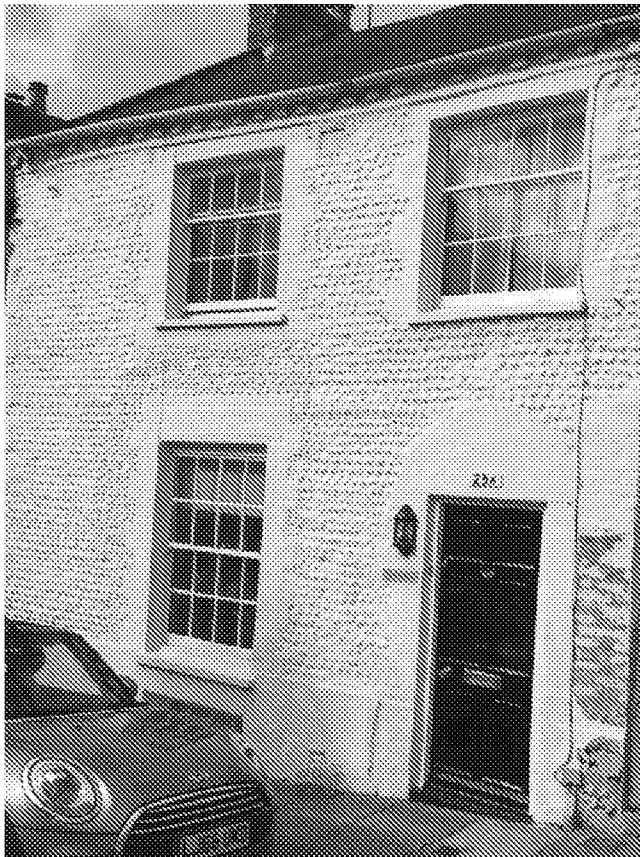
25a King Street, adjoining property to the south.
