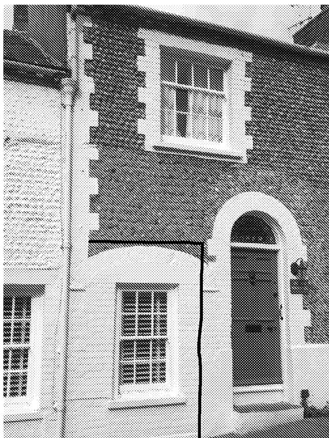
The Old Bakehouse – property adjoining to the north
