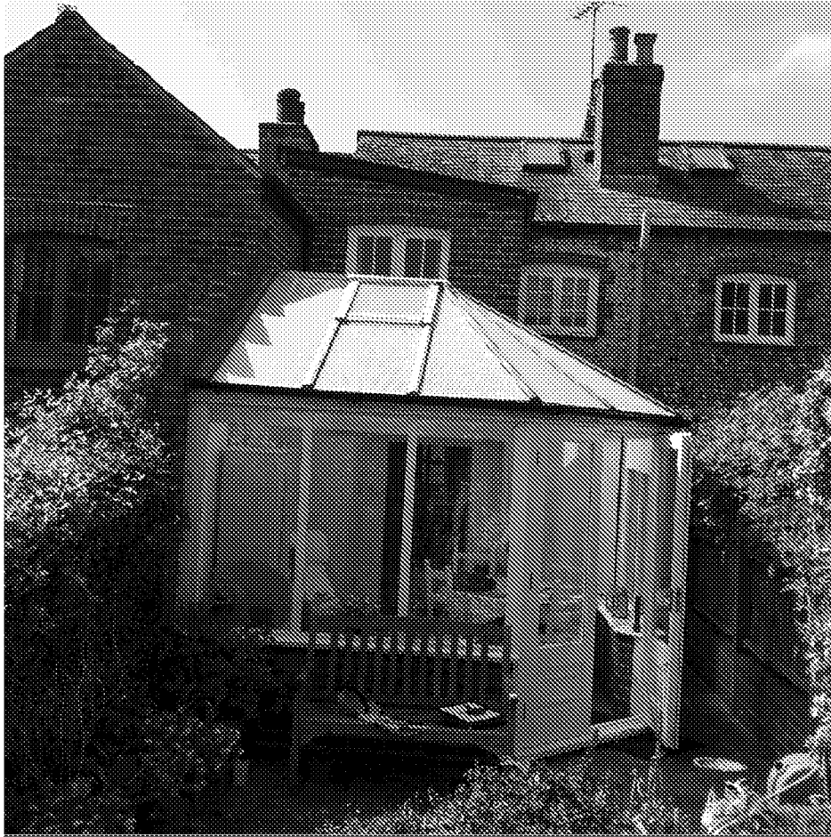
EXISTING CONSERVATORY TO REAR
