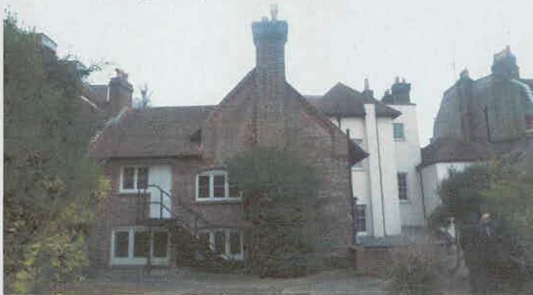
Photograph of existing rear of building
