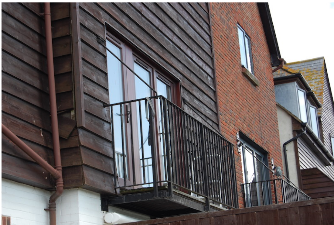
figure 1 Balcony to flat 3
