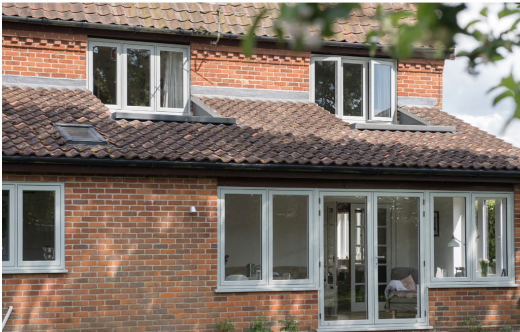
figure 3 Typical Residence 7 French doors and windows
