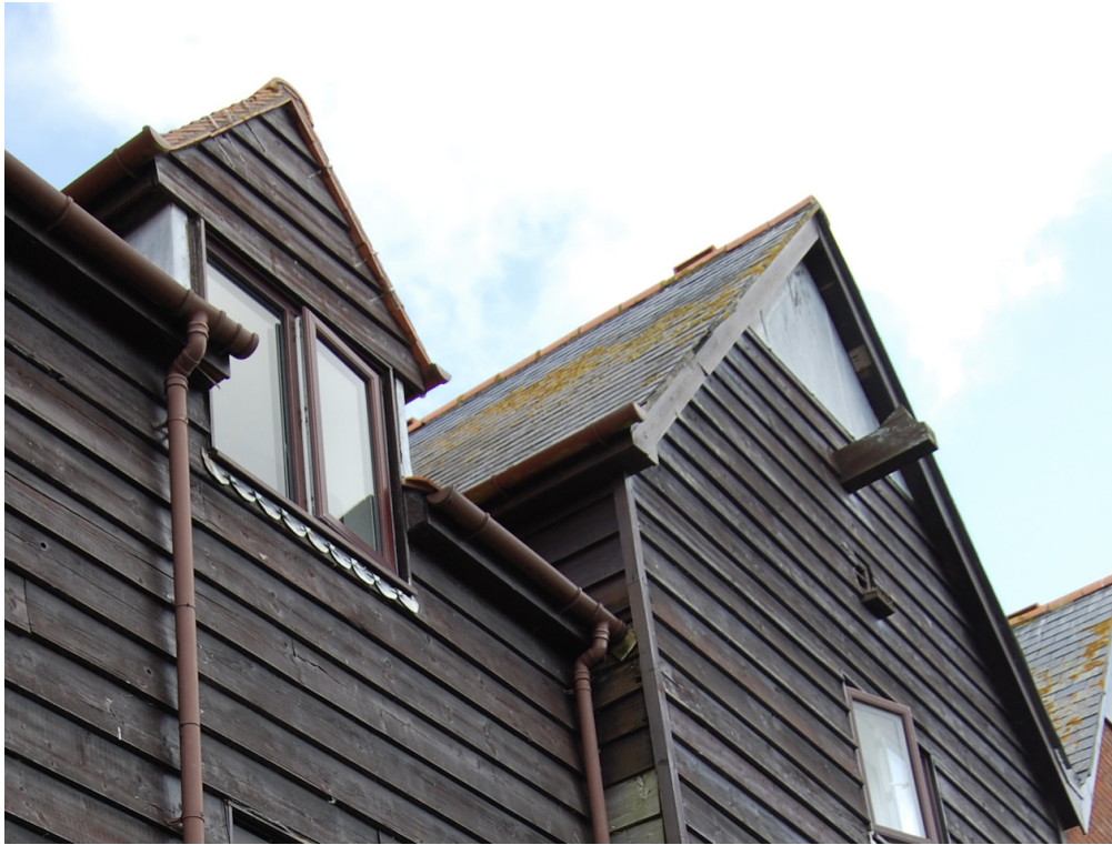
figure 2 Replacement windows flat 5
